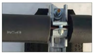
Aeroflex USA recommends Aerofix<sup>®</sup> insulated pipe supports to provide a hermetic system of AEROFLEX® EPDM closed cell elastomeric insulation through strut clamps to ultimately prevent a thermal break, energy loss and corrosion under insulation.
